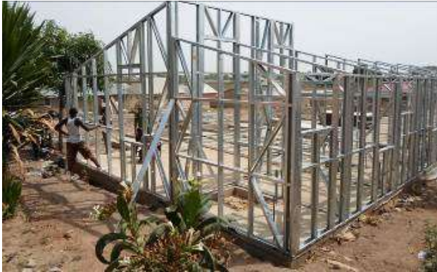
Dry wall construction by Nigerite/ Etex Group
