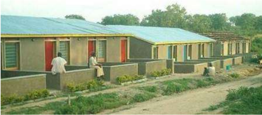
The Fuller Housing Estate, Luvu showing blocks of 4 units
